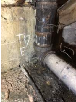
Photo 3-17a: Truss 17 East Bearing North Face
