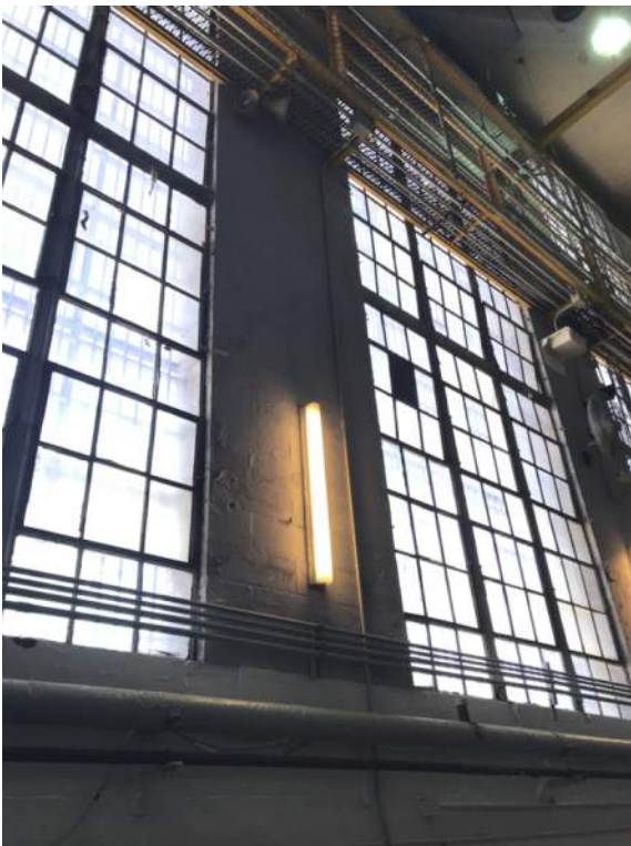
Photo 1-1g: Masonry Interior face of east pier
