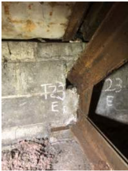
Photo 3-23a: Truss 23 East Bearing North Face
