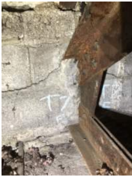
Photo 3-7a: Truss 7 East Bearing North Face
