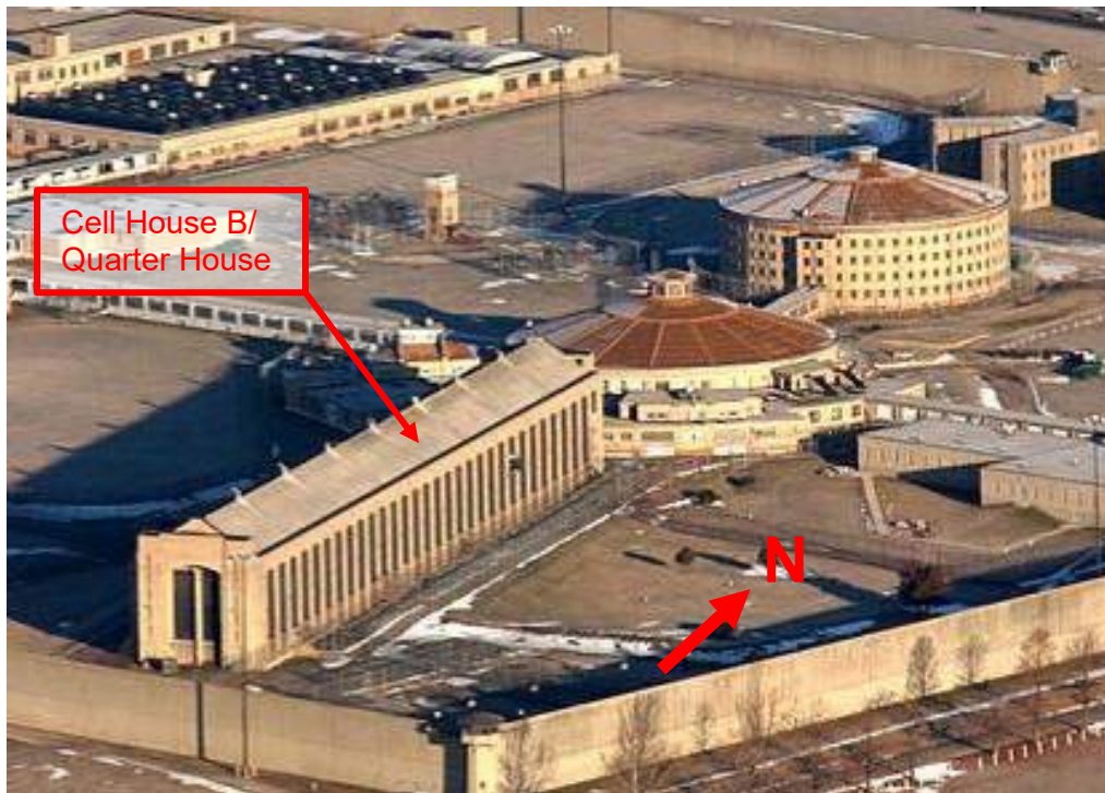
Fig. 1 View of Cell House B/Quarter House.
