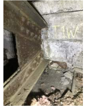
Photo 3-1d: Truss 1 West Bearing North Face
