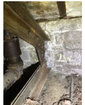
Photo 3-2d: Truss 2 West Bearing North Face
