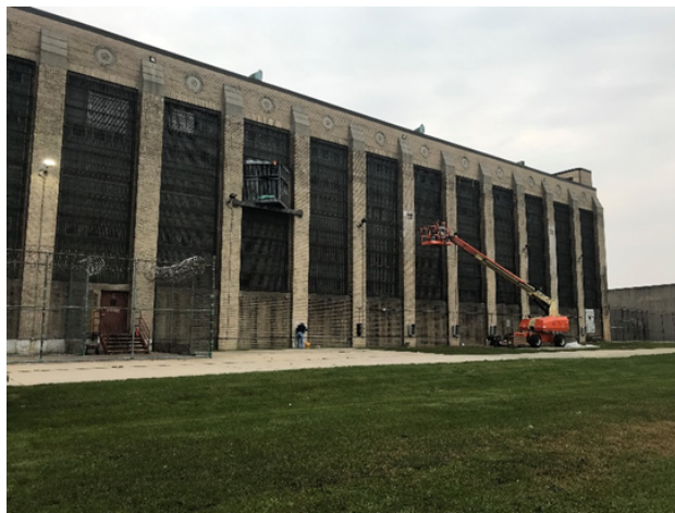
Figure 3: West wall looking south
