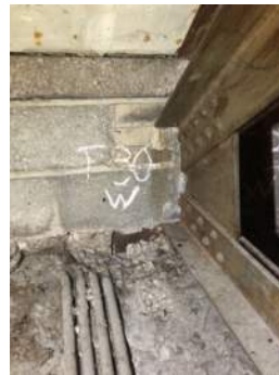
Photo 3-30c: Truss 30 West Bearing South Face
