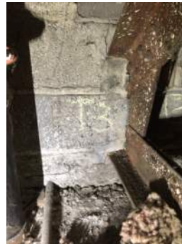
Photo 3-3c: Truss 3 West Bearing South Face
