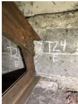
Photo 3-24b: Truss 24 East Bearing South Face
