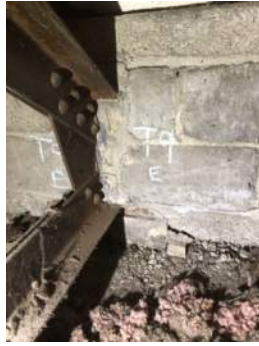
Photo 3-9b: Truss 9 East Bearing South Face
