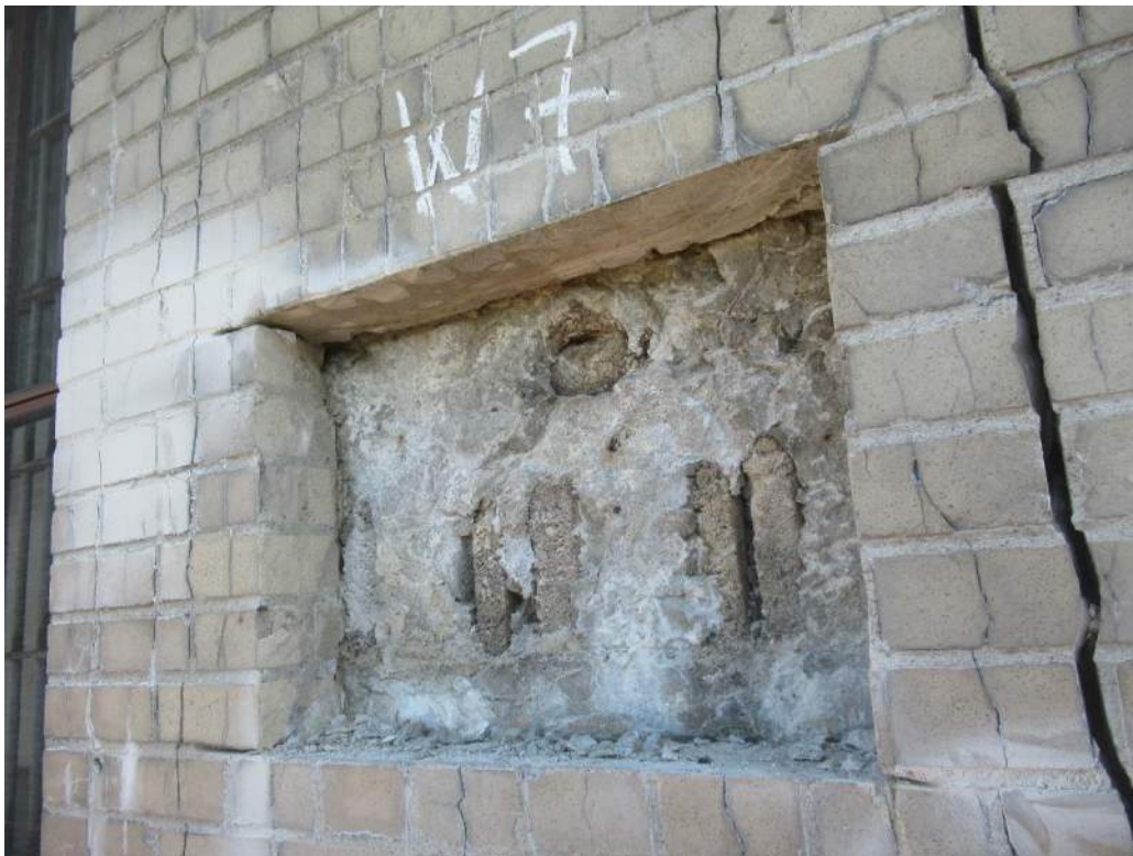
Fig. 17 Pier W7 exterior opening at ~24 ft.
