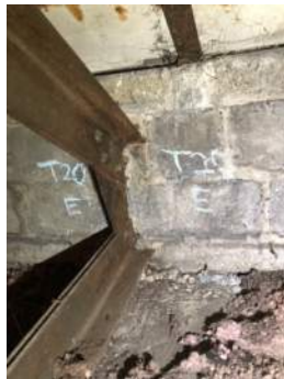
Photo 3-20b: Truss 20 East Bearing South Face
