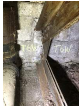
Photo 3-6c: Truss 6 West Bearing South Face
