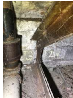
Photo 3-2c: Truss 2 West Bearing South Face
