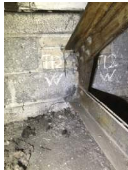
Photo 3-12c: Truss 12 West Bearing South Face
