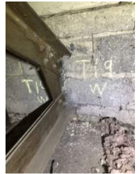
Photo 3-19d: Truss 19 West Bearing North Face
