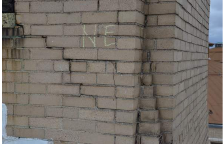
Photo 1-2k: Masonry NE Gable Wall
