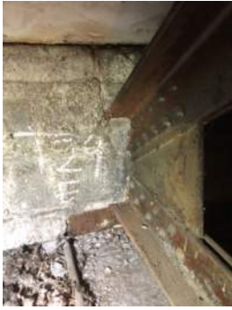
Photo 3-29a: Truss 29 East Bearing North Face
