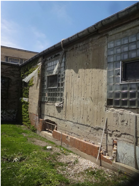
Typical location, removed masonry at grade.
