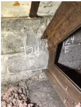
Photo 3-24a: Truss 24 East Bearing North Face
