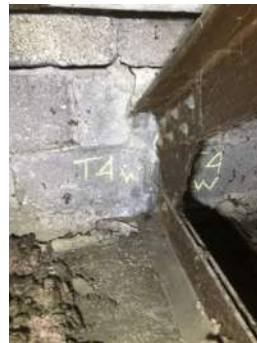
Photo 3-4c: Truss 4 West Bearing South Face
