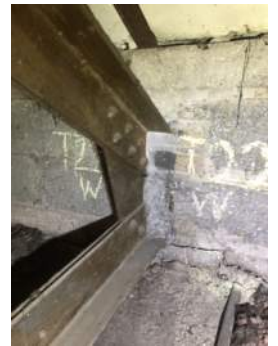
Photo 3-22d: Truss 22 West Bearing North Face
