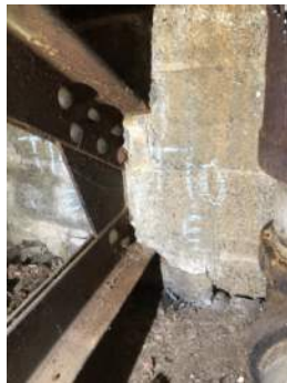
Photo 3-10b: Truss 10 East Bearing South Face
