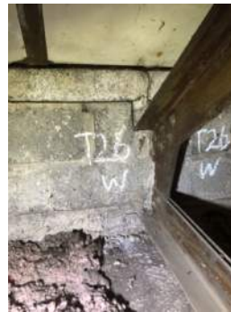
Photo 3-26c: Truss 26 West Bearing South Face
