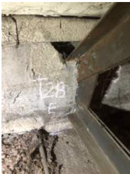
Photo 3-28a: Truss 28 East Bearing North Face
