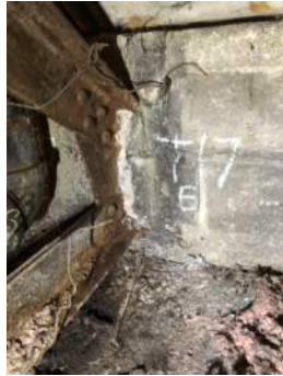
Photo 3-17b: Truss 17 East Bearing South Face
