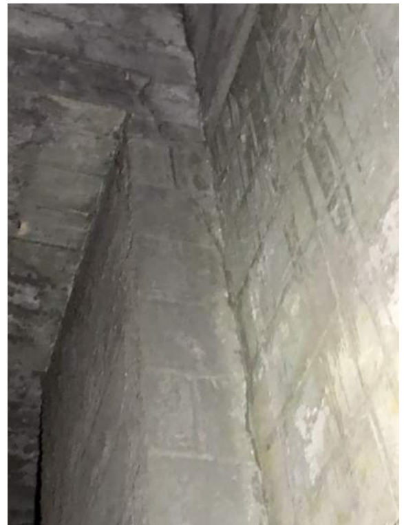
Photo 1-3m: Masonry North Arch Interior View
