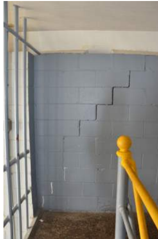
Photo 2-21: Interior Stair Landing wall
