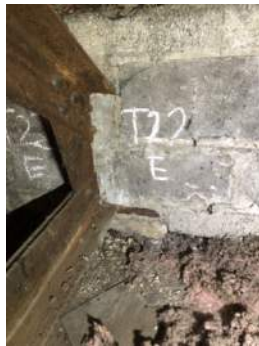
Photo 3-22b: Truss 22 East Bearing South Face
