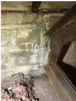
Photo 3-10a: Truss 10 East Bearing North Face
