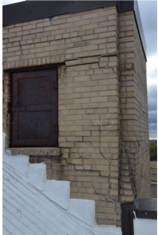
Photo 1-2g: Masonry SW Gable Wall
