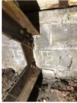
Photo 3-5b: Truss 5 East Bearing South Face
