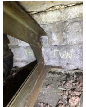
Photo 3-6d: Truss 6 West Bearing North Face
