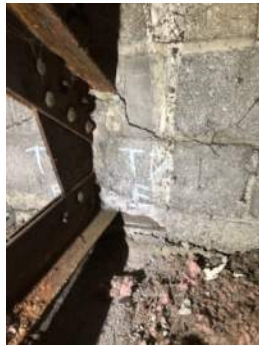
Photo 3-7b: Truss 7 East Bearing South Face
