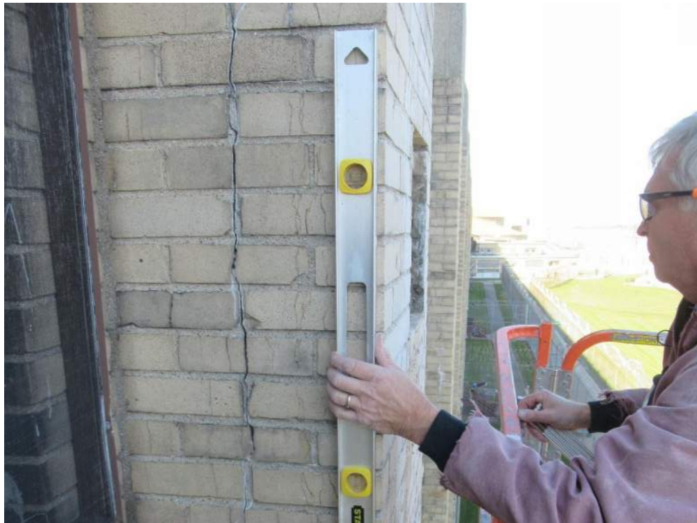
Fig. 15 Pier E2 south return brick face at ~36 ft.
