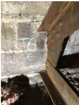
Photo 3-6a: Truss 6 East Bearing North Face
