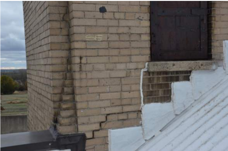
Photo 1-2h: Masonry SE Gable Wall
