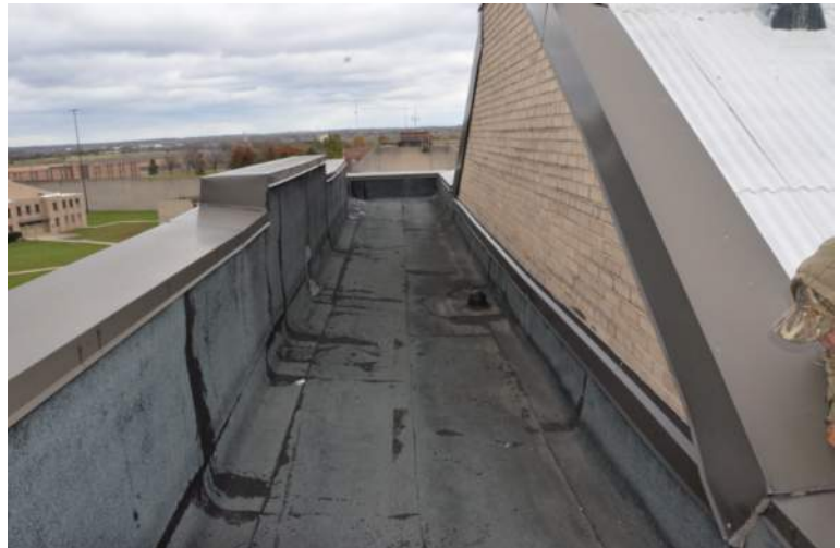
Photo 1-2i: Masonry South Gable Wall
