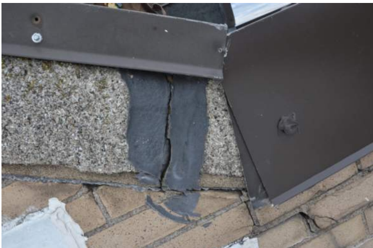
Photo 1-6c: Masonry South Gable wall Coping
