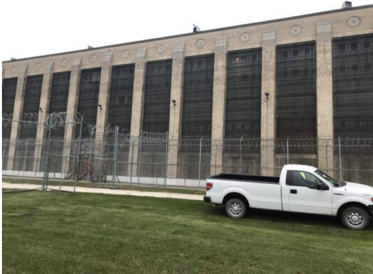
Photo 1-1a: Masonry West Elevation
