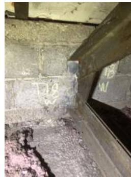
Photo 3-18c: Truss 18 West Bearing South Face
