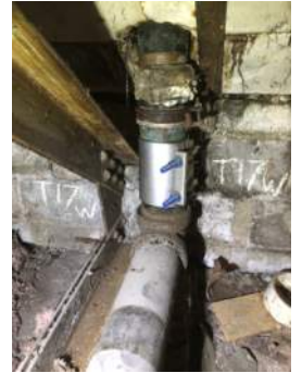
Photo 3-17d: Truss 17 West Bearing North Face
