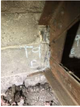
Photo 3-9a: Truss 9 East Bearing North Face
