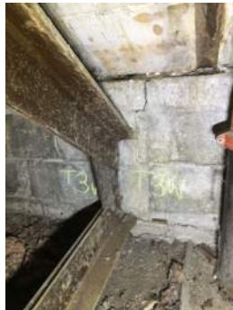
Photo 3-3b: Truss 3 East Bearing South Face
