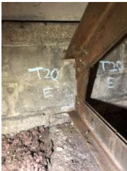
Photo 3-20a: Truss 20 East Bearing North Face
