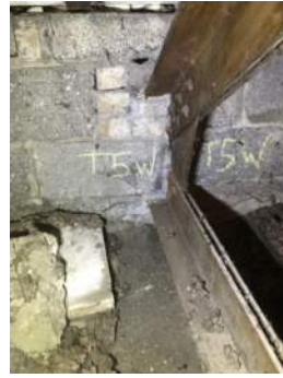
Photo 3-5c: Truss 5 West Bearing South Face
