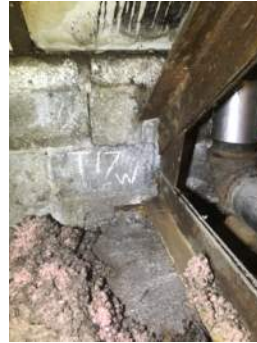
Photo 3-17c: Truss 17 West Bearing South Face
