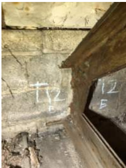
Photo 3-12a: Truss 12 East Bearing North Face
