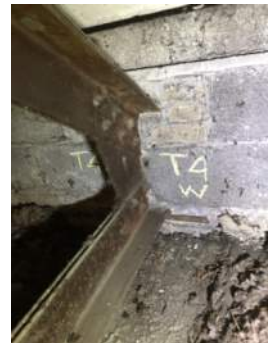
Photo 3-4d: Truss 4 West Bearing North Face
