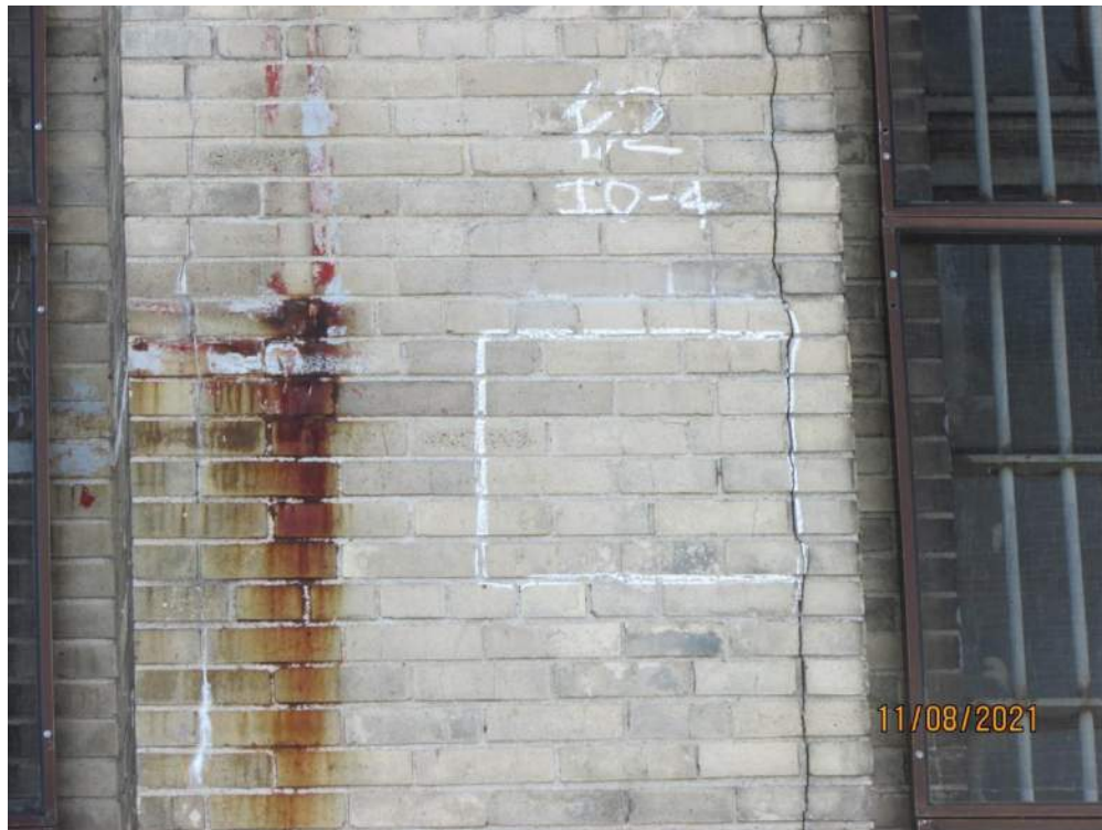
Fig. 13 Pier E2 front brick face at ~ 18 ft.
