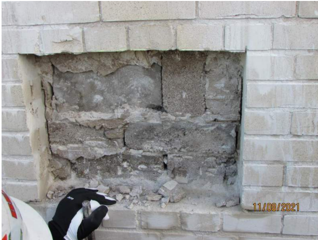
Fig. 18 Pier W9 exterior opening at ~4 ft.
