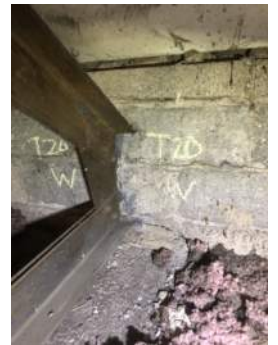
Photo 3-20d: Truss 20 West Bearing North Face
