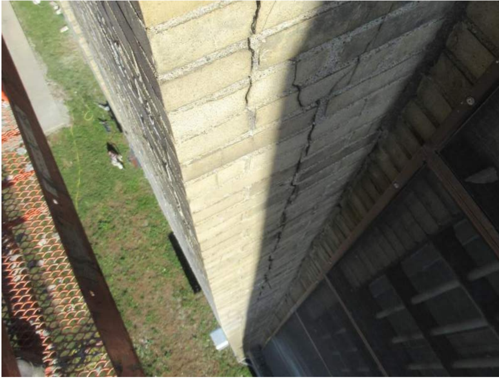
Fig. 10 Pier W7 south return brick face at ~24 ft.
