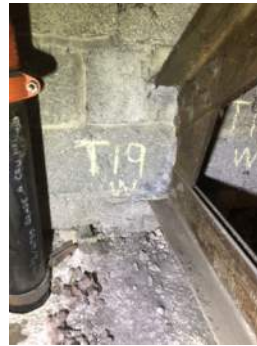
Photo 3-19c: Truss 19 West Bearing South Face
