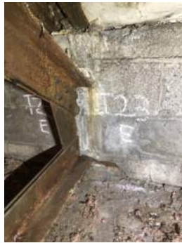
Photo 3-23b: Truss 23 East Bearing South Face
