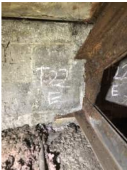
Photo 3-22a: Truss 22 East Bearing North Face
