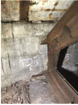
Photo 3-25a: Truss 25 East Bearing North Face
