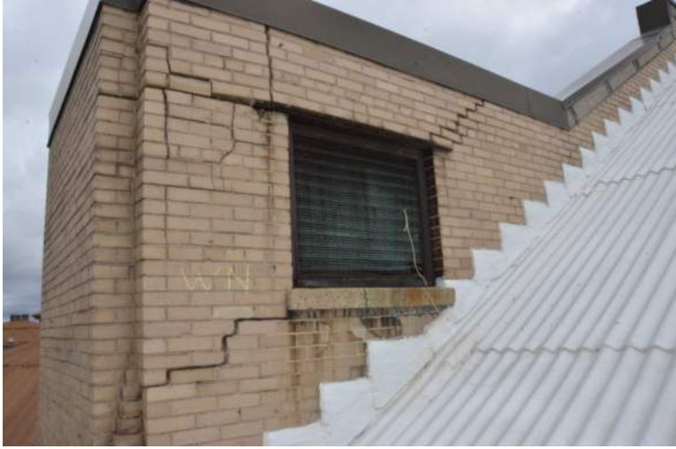
Photo 1-6a: Masonry New roofing over Main Roof
