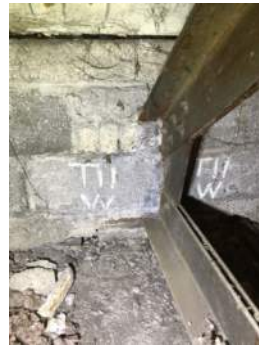
Photo 3-11c: Truss 11 West Bearing South Face
