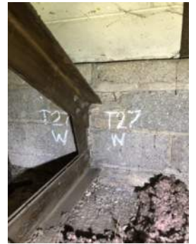
Photo 3-27d: Truss 27 West Bearing North Face
