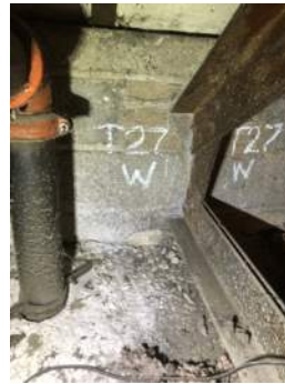
Photo 3-27c: Truss 27 West Bearing South Face
