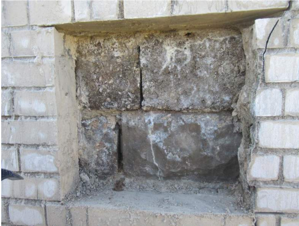
Fig. 20 Pier E2 exterior opening at ~36 ft.
