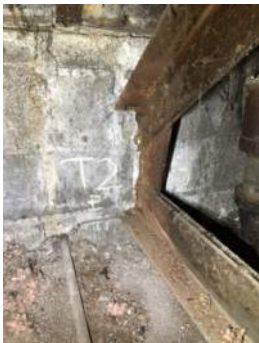
Photo 3-2a: Truss 2 East Bearing North Face
