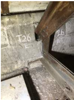
Photo 3-26a: Truss 26 East Bearing North Face
