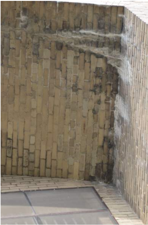
Photo 1-3d: Masonry South Arch East Corner
