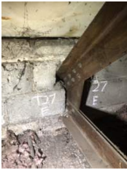
Photo 3-27a: Truss 27 East Bearing North Face
