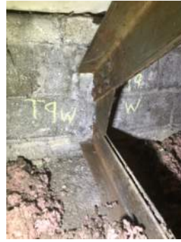
Photo 3-9c: Truss 9 West Bearing South Face
