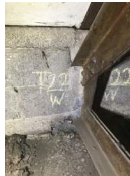
Photo 3-22c: Truss 22 West Bearing South Face
