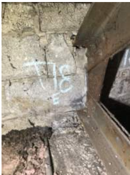
Photo 3-18a: Truss 18 East Bearing North Face
