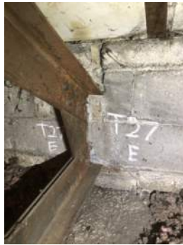
Photo 3-27b: Truss 27 East Bearing South Face
