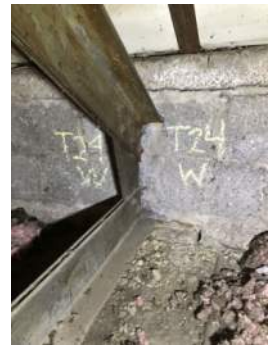
Photo 3-24d: Truss 24 West Bearing North Face
