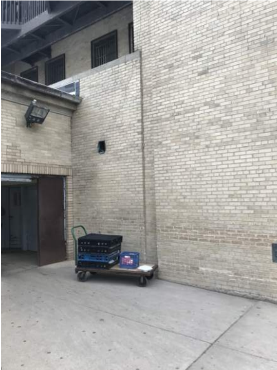
Photo 1-2f: Masonry NW corner
