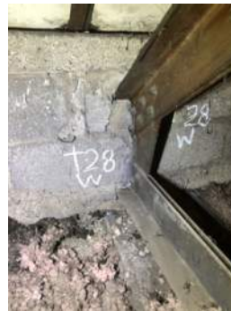
Photo 3-28c: Truss 28 West Bearing South Face
