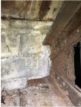
Photo 3-1a: Truss 1 East Bearing North Face
