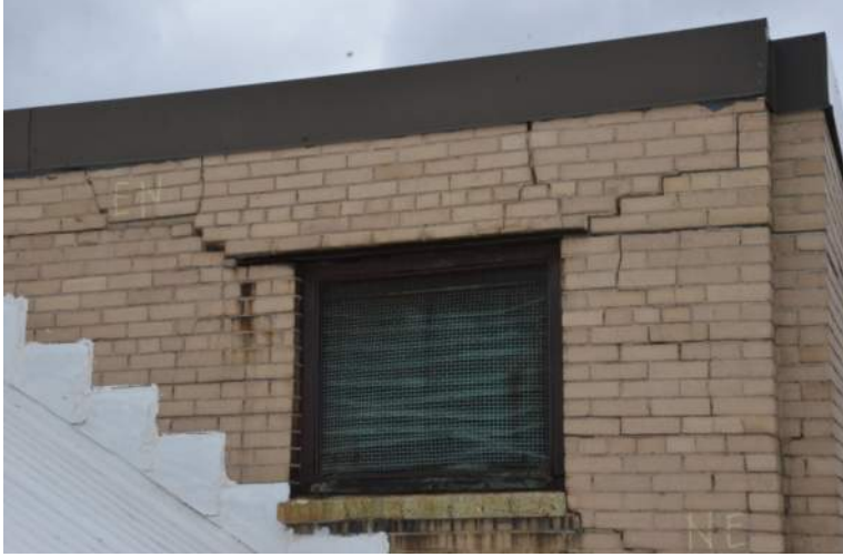
Photo 1-2j: Masonry NE Gable Wall
