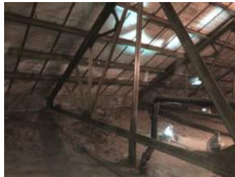
Photo 3-32: Attic North End View of east side of Truss 30 and roof
