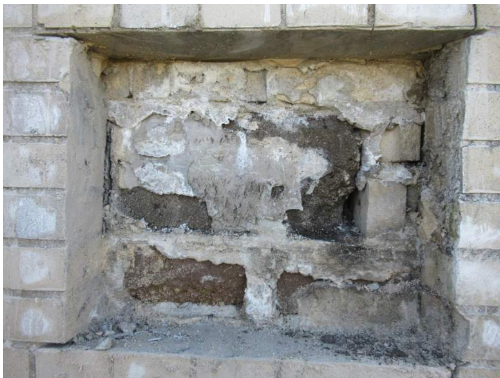
Fig. 19 Pier E2 exterior opening at ~18 ft.
