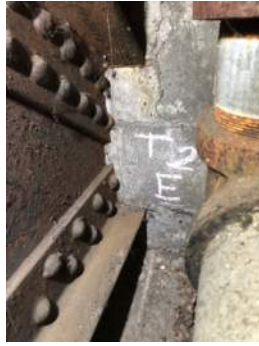
Photo 3-29b: Truss 29 East Bearing South Face
