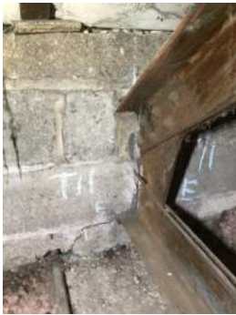
Photo 3-11a: Truss 11 East Bearing North Face
