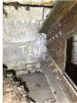
Photo 3-1c: Truss 1 West Bearing South Face
