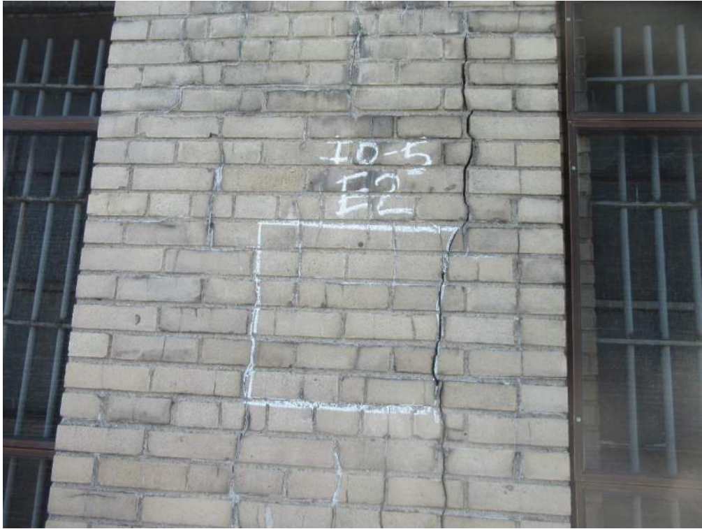
Fig. 14 Pier E2 front brick face at ~ 36 ft.
