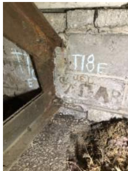
Photo 3-18b: Truss 18 East Bearing South Face
