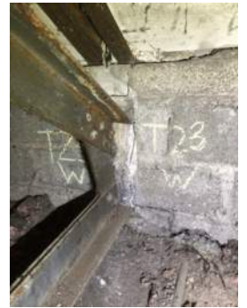
Photo 3-23d: Truss 23 West Bearing North Face
