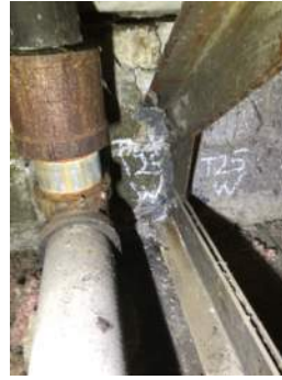
Photo 3-25c: Truss 25 West Bearing South Face
