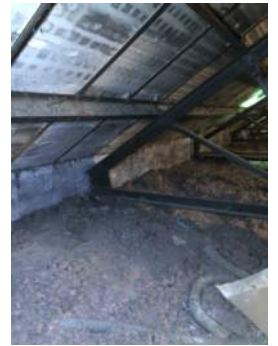
Photo 3-34: Attic South End View of west side of Truss 1 and roof
