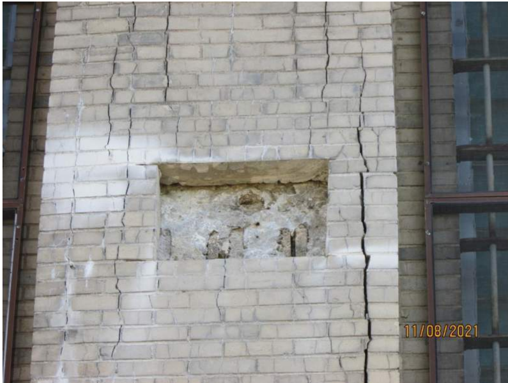
Fig. 8 Pier W7 front brick face at ~24 ft.
