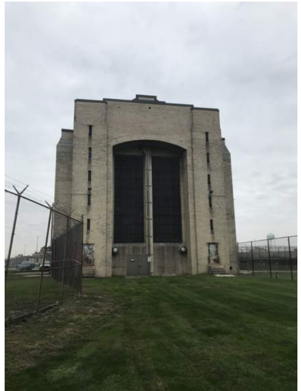
Photo 1-3a: Masonry South Arch Elevation
