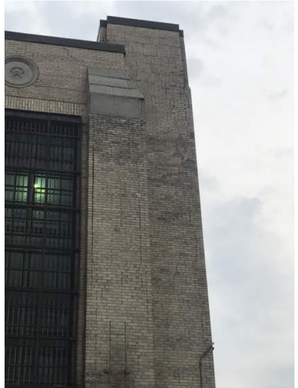
Photo 1-2c: Masonry SW corner
