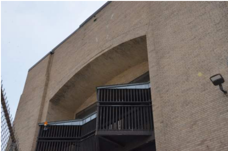
Photo 1-3h: Masonry North Arch
