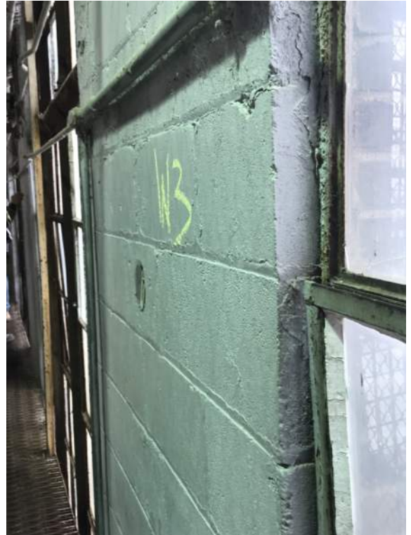
Photo 1-1f: Masonry Interior face of Pier W3
