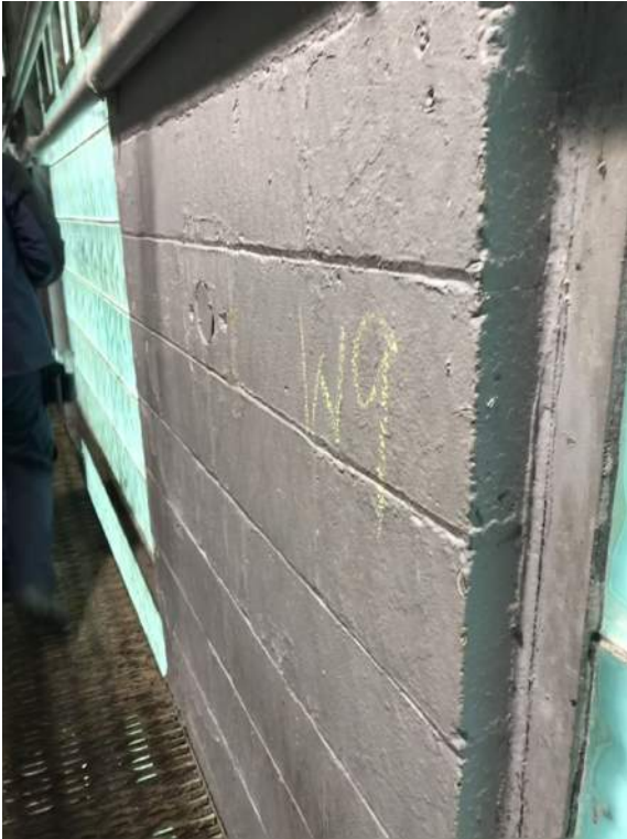
Photo 1-1e: Masonry Interior face of Pier W9
