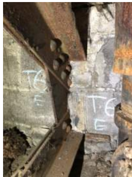
Photo 3-6b: Truss 6 East Bearing South Face
