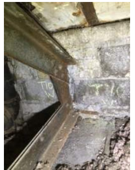
Photo 3-10d: Truss 10 West Bearing North Face
