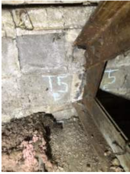
Photo 3-5a: Truss 5 East Bearing North Face
