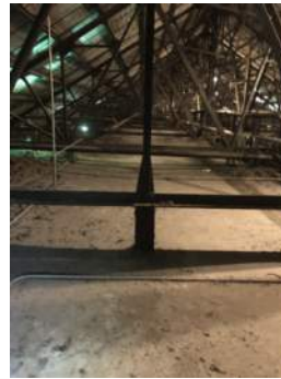
Photo 3-33: Attic South End looking North at Truss 1 with ceiling hanger
