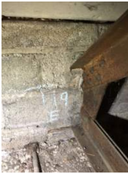
Photo 3-19a: Truss 19 East Bearing North Face
