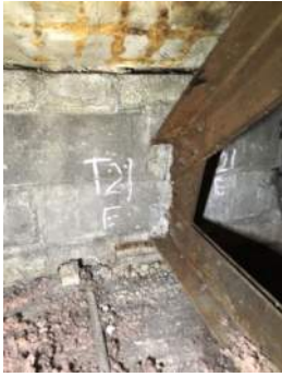
Photo 3-21a: Truss 21 East Bearing North Face
