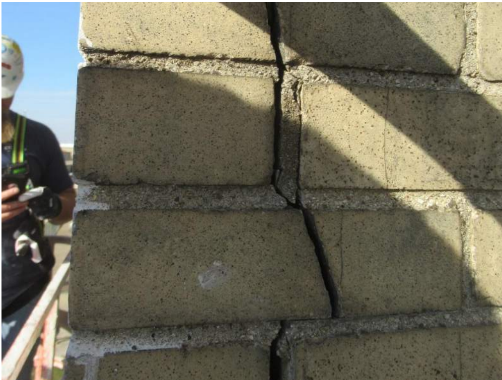
Fig. 7 Pier W3 south return brick face at ~30 ft.
