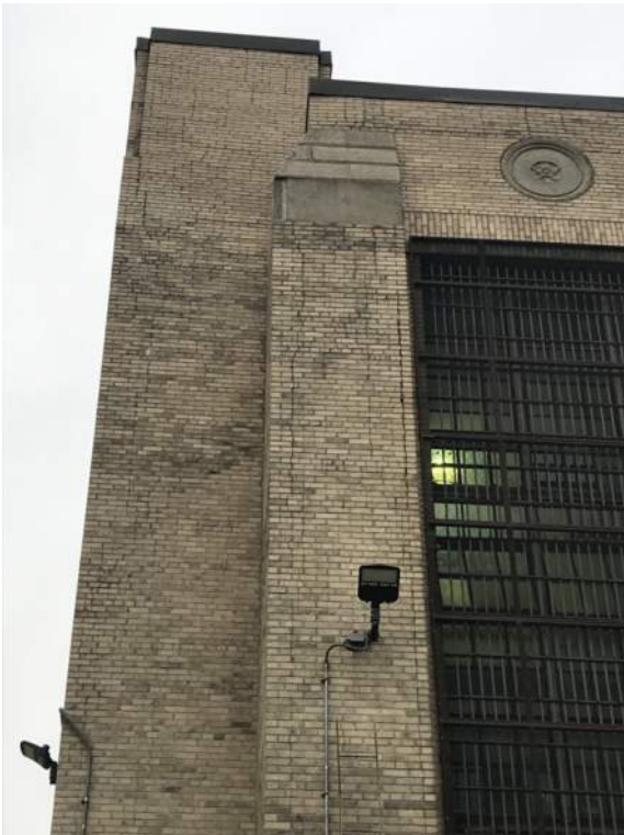
Photo 1-2d: Masonry SE corner
