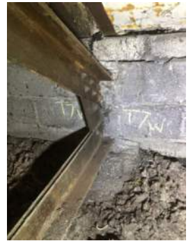
Photo 3-7d: Truss 7 West Bearing North Face
