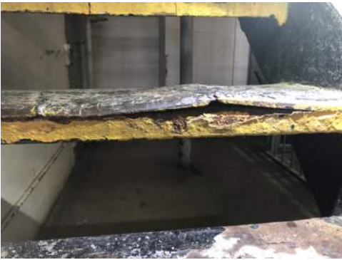
Photo 2-20b: Interior Steel stairs
