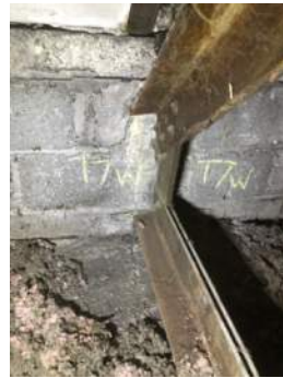
Photo 3-7c: Truss 7 West Bearing South Face
