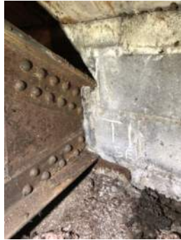
Photo 3-1b: Truss 1 East Bearing South Face
