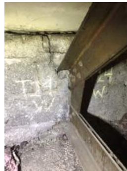
Photo 3-24c: Truss 24 West Bearing South Face
