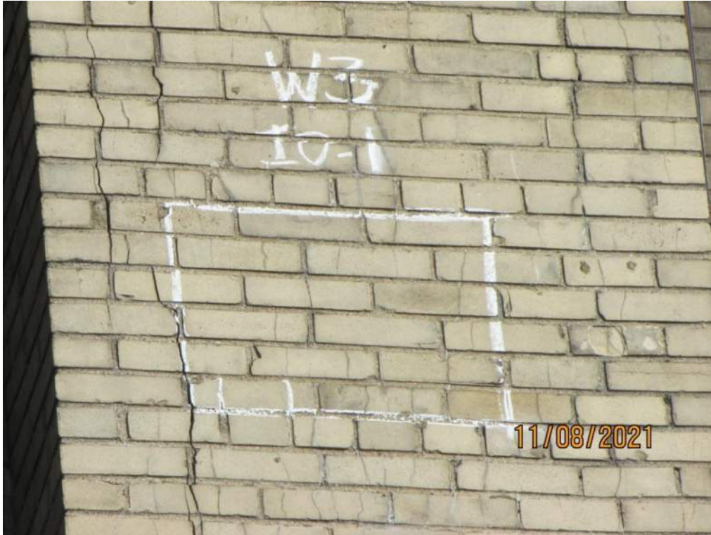
Fig. 6 Pier W3 front brick face at ~30 ft.
