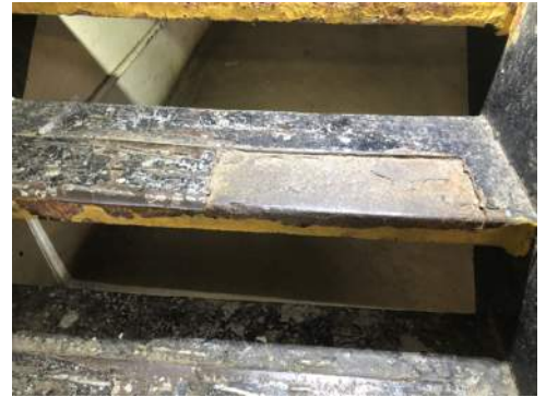
Photo 2-20a: Interior Steel stairs
