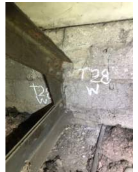
Photo 3-28d: Truss 28 West Bearing North Face
