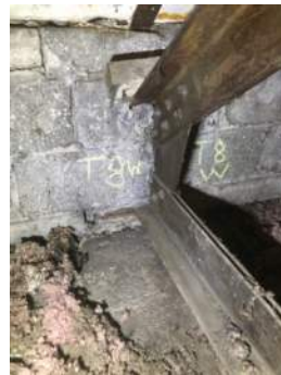
Photo 3-8c: Truss 8 West Bearing South Face
