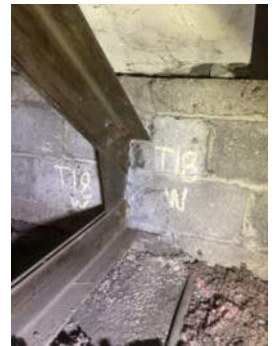
Photo 3-18d: Truss 18 West Bearing North Face
