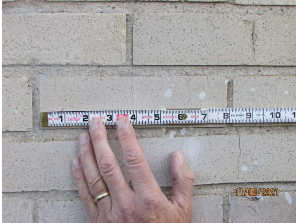
Fig. 12 Pier W9 front brick face at ~4 ft.
