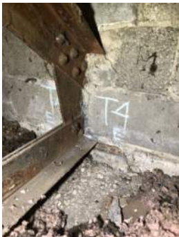
Photo 3-4a: Truss 4 East Bearing North Face
