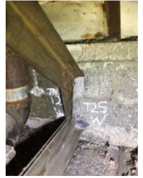
Photo 3-25d: Truss 25 West Bearing North Face
