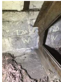
Photo 3-20c: Truss 20 West Bearing South Face
