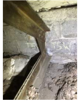
Photo 3-5d: Truss 5 West Bearing North Face
