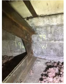
Photo 3-9d: Truss 9 West Bearing North Face
