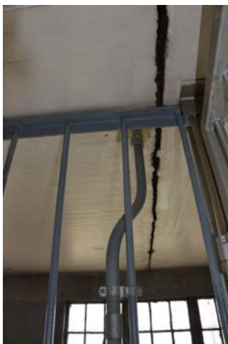
Photo 2-6: Interior Ceiling Slab Joint east to west
