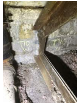
Photo 3-10c: Truss 10 West Bearing South Face
