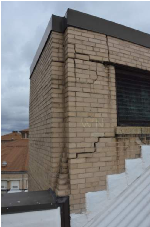
Photo 1-2l: Masonry NW Gable Wall
