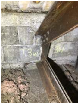
Photo 3-3a: Truss 3 East Bearing North Face
