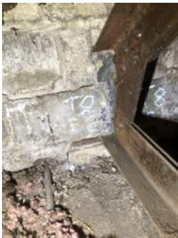
Photo 3-8a: Truss 8 East Bearing North Face
