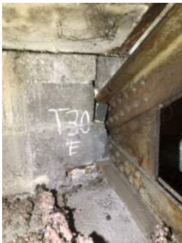
Photo 3-30a: Truss 30 East Bearing North Face
