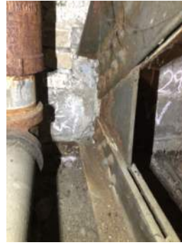
Photo 3-29c: Truss 29 West Bearing South Face
