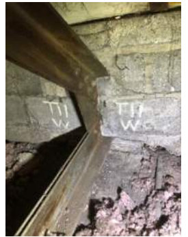
Photo 3-11d: Truss 11 West Bearing North Face
