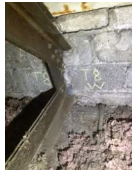
Photo 3-8d: Truss 8 West Bearing North Face
