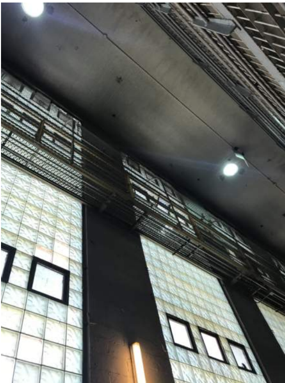
Photo 1-5g West Wall Glass Block Windows
