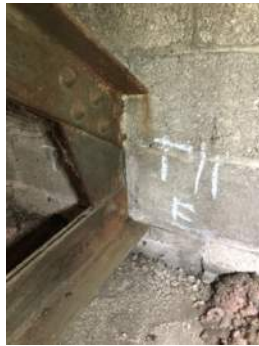
Photo 3-11b: Truss 11 East Bearing South Face
