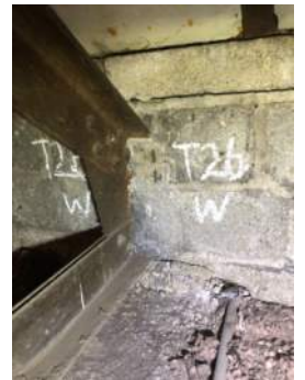
Photo 3-26d: Truss 26 West Bearing North Face
