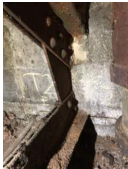
Photo 3-2b: Truss 2 East Bearing South Face
