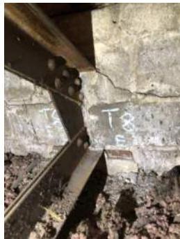
Photo 3-8b: Truss 8 East Bearing South Face
