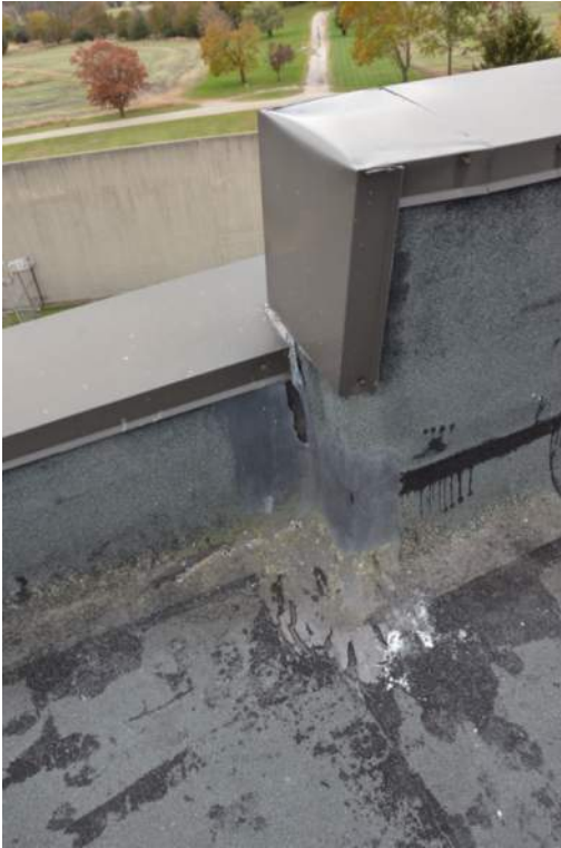
Photo 1-7b: Masonry South End Bay Roof and Arch Coping
