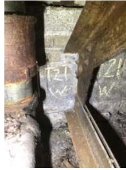
Photo 3-21c: Truss 21 West Bearing South Face
