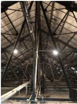
Photo 3-31 Attic North End looking south from Truss 30
