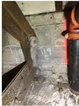
Photo 3-19b: Truss 19 East Bearing South Face
