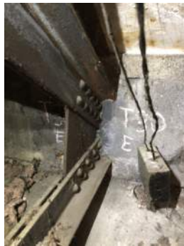
Photo 3-30b: Truss 30 East Bearing South Face
