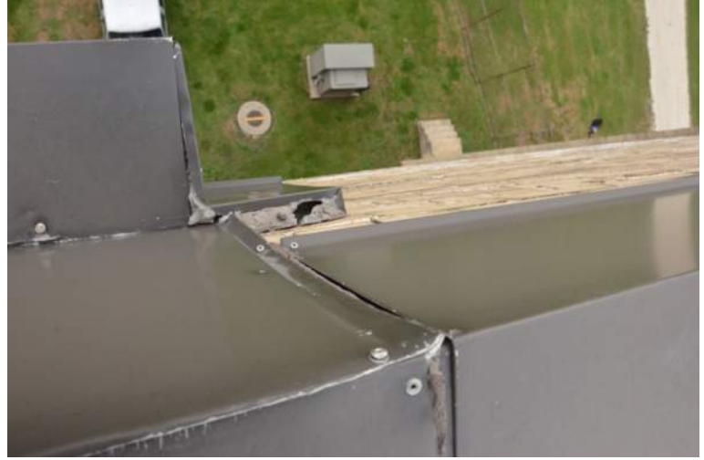
Photo 1-6b: Masonry South elevation Coping 1
