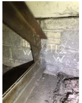
Photo 3-12d: Truss 12 West Bearing North Face
