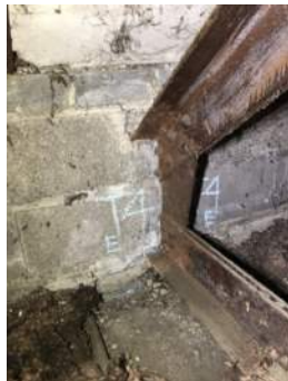
Photo 3-4b: Truss 4 East Bearing South Face
