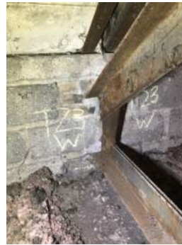
Photo 3-23c: Truss 23 West Bearing South Face
