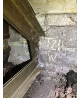
Photo 3-21d: Truss 21 West Bearing North Face
