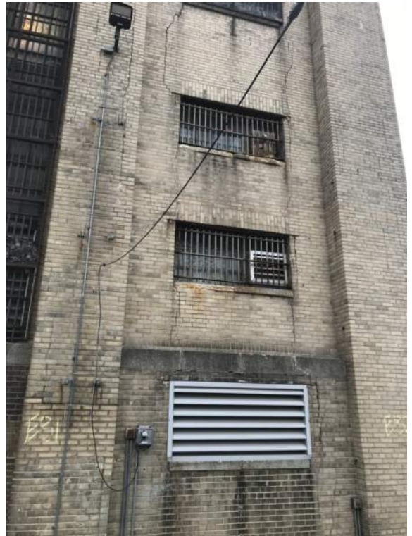
Photo 1-2e: Masonry NE corner
