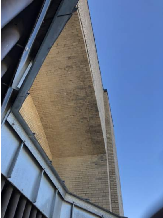
Photo 1-3j: Masonry North Arch
