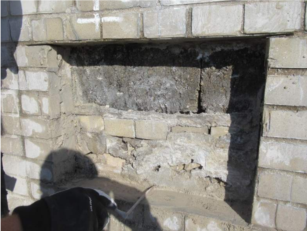
Fig. 16 Pier W3 exterior opening at ~30 ft.
