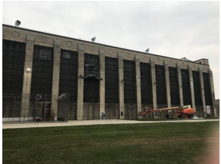
Photo 1-1b: Masonry West elevation - 3 test openings
