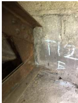
Photo 3-12b: Truss 12 East Bearing South Face
