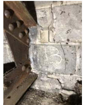
Photo 3-3d: Truss 3 West Bearing North Face
