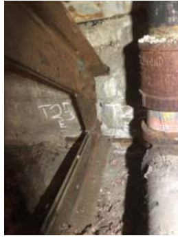
Photo 3-25b: Truss 25 East Bearing South Face
