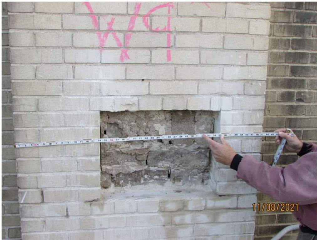
Fig. 11 Pier W9 front brick face at ~4 ft.
