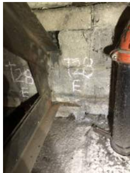
Photo 3-28b: Truss 28 East Bearing South Face
