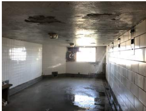
Photo 2-16: Interior B House shower ceiling/ E House shower floor
