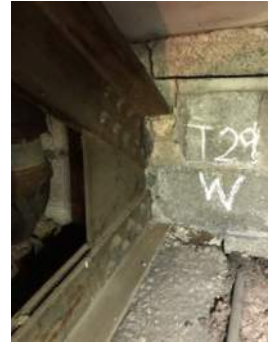
Photo 3-29d: Truss 29 West Bearing North Face
