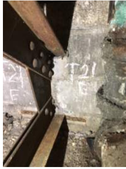
Photo 3-21b: Truss 21 East Bearing South Face
