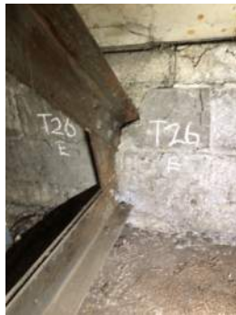
Photo 3-26b: Truss 26 East Bearing South Face
