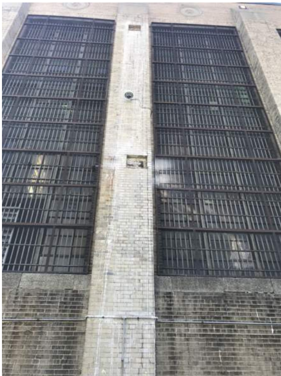
Photo 1-1c: Masonry Pier E2 - 2 test openings
