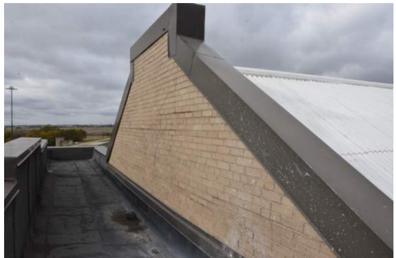
Photo 1-7a: Masonry South End Bay Roof
