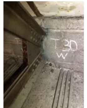
Photo 3-30d: Truss 30 West Bearing North Face
