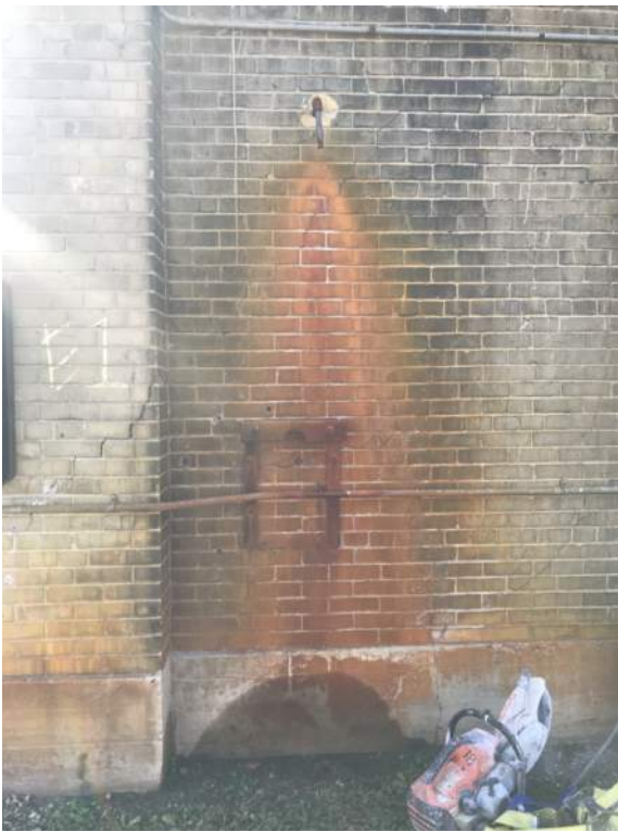
Photo 1-8b: Condensate at SW corner local settlement
