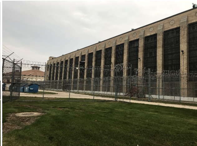
Figure 4: West wall looking north
